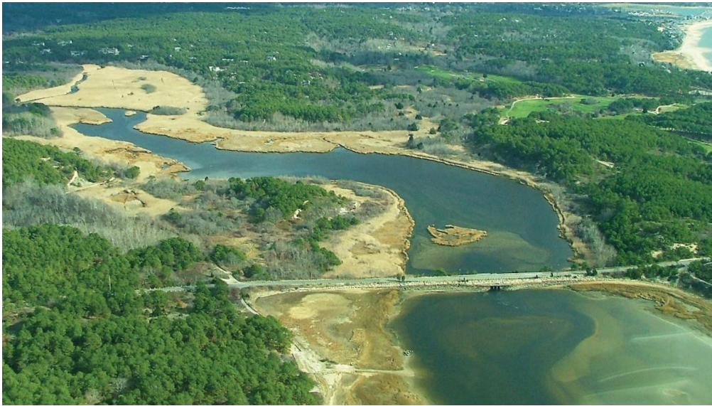
Restoring the estuary's tidal flows hinge on replacing the 1908 dike with a new bridge and two secondary dikes. With strong partnerships and funding, we hope to start construction in 2018. © Friends of Herring River.
